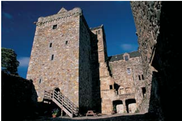
The tower with an original entrance in the west wall, the new stair turret and the east range with ground floor loggia (open arcade) © Clackmannanshire Council
